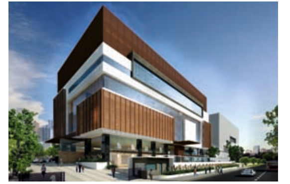
SMR VINAY METRO MALL & MULTIPLEX, MIYAPUR
